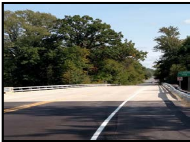
East Michigan Avenue Bridge, Charleston Township
