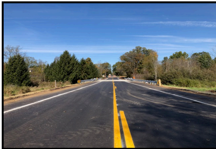
36th Street - over Dorrance Creek, Climax Township
