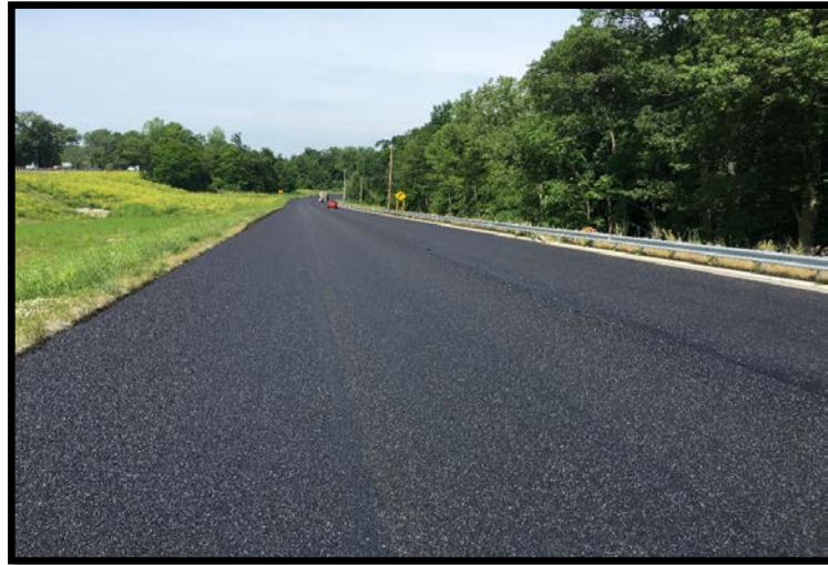
East Michigan Avenue west of 40th Street, Charleston Township
